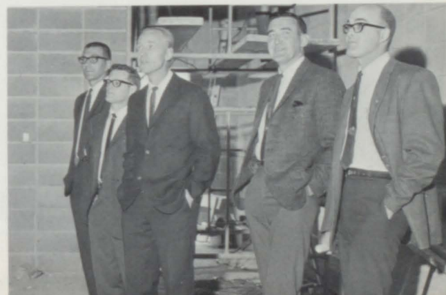
School board members view the early stages of construction on the new addition.
